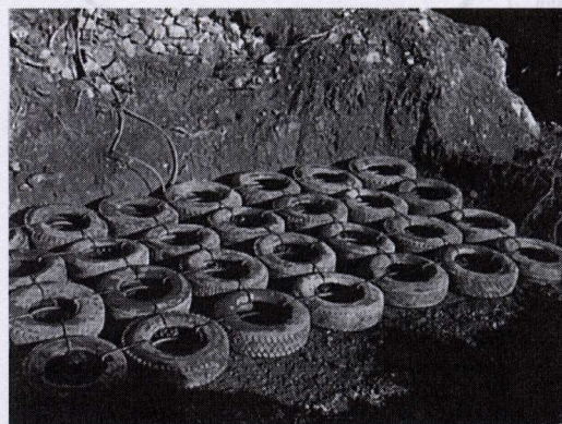
Photo n°4: Reduce active earth pressure with trucks tyres
